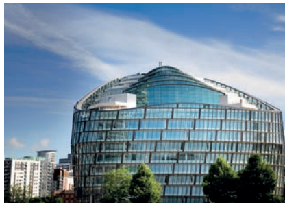
Co-operative Group Headquarters, UK
